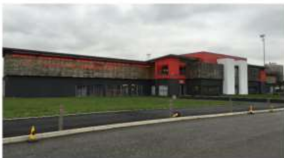
Home Stadium Broadhurst Park 6.5 Million £ Investment by Own Finance
